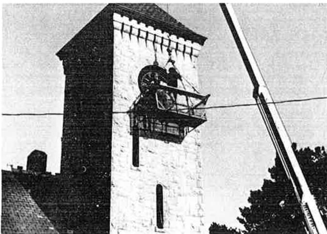
Workmen insert new faces into the clock tower, September 1987.
