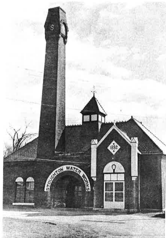
Stoughton Water Works
