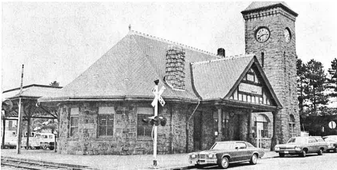
Stoughton Railroad Station today
