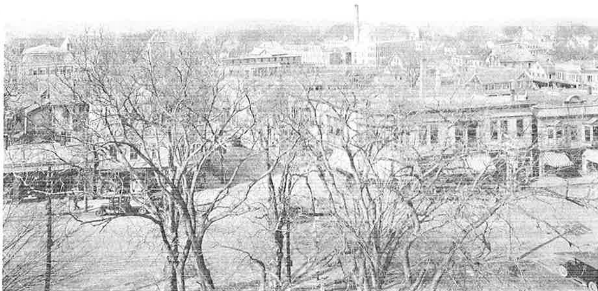
General View, showing Stoughton Rubber Co.
